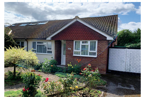
↓ The property as it is today. Janis and Dave would like to convert the loft and add a rear-and-side extension to maximise the available floor area.
